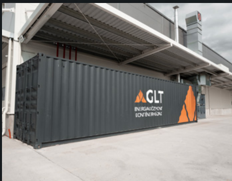
water/water heatpump center
